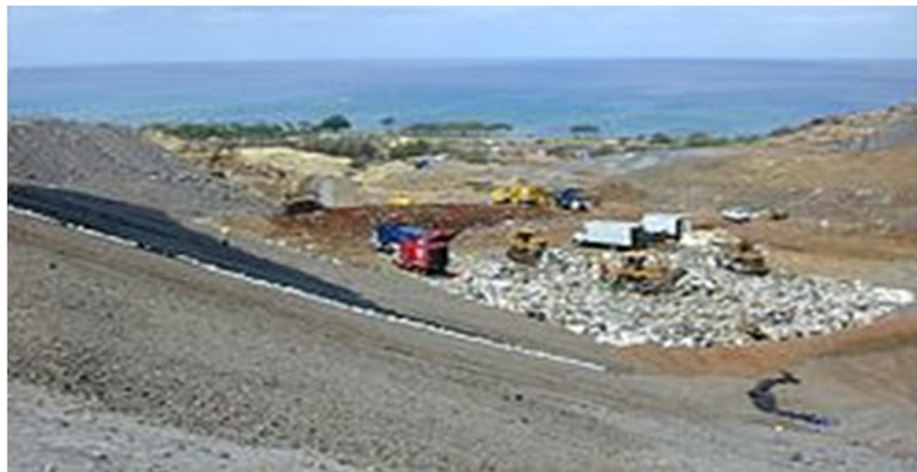
Figure 2: Landfill operation in Hawaii. Note that the area being filled is a single, well-defined "cell" and that a rubberized landfill liner is in place (exposed on the left) to prevent contamination by leachates migrating downward through the underlying geological formation.
